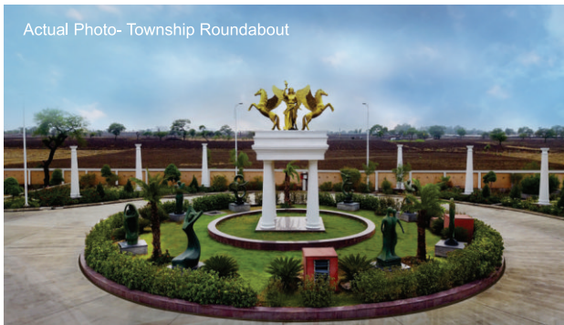
Actual Photo- Township Shops/ Offices
